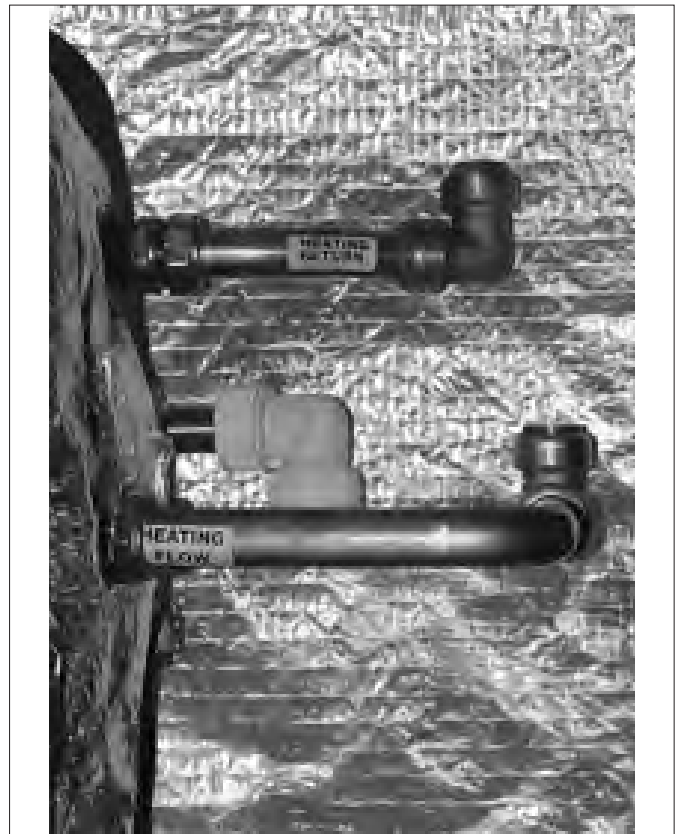
Figure 5-1: Non system boiler flow and return connections
