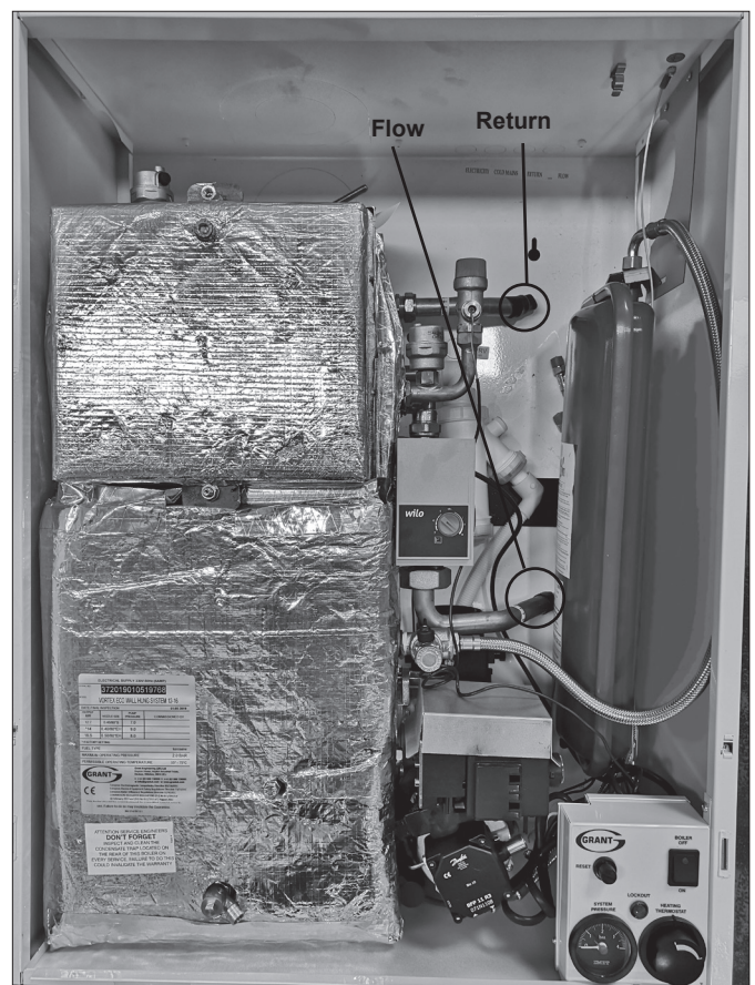
Figure 5-2: System boiler flow and return connections
