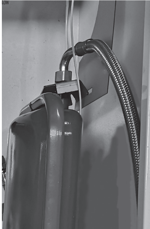
Figure 4-3: Expansion vessel, Expansion vessel bracket and hose connection - System model only
