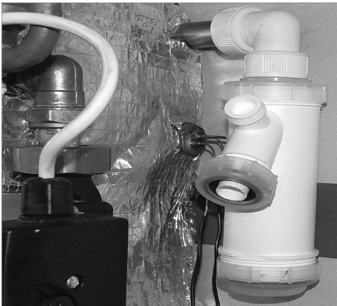
Figure 6-2: Condensate trap location
